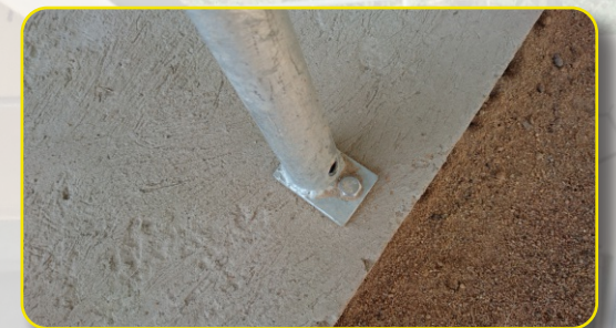
Feet firmly bolted to deck.
