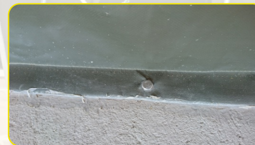
PVC splashguard bolted to deck and sealed
